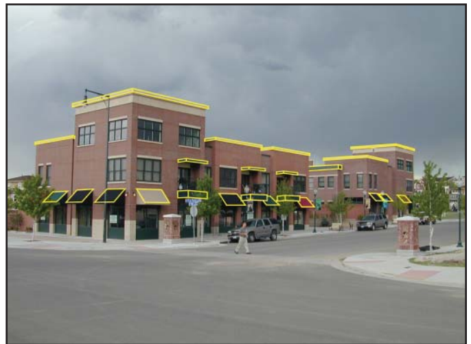
Articulation is how the elements of a form come together to shape exterior space. In this photo, articulation is displayed by the arrangement and variations in the streetscape and building which help form people-oriented spaces.
