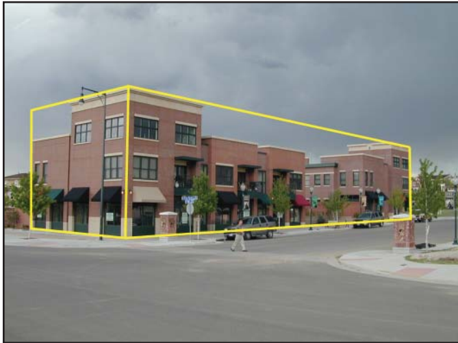
Mass is the overall volume of a building. Mass is the roughest scale of how a block face equals its aggregate size.
