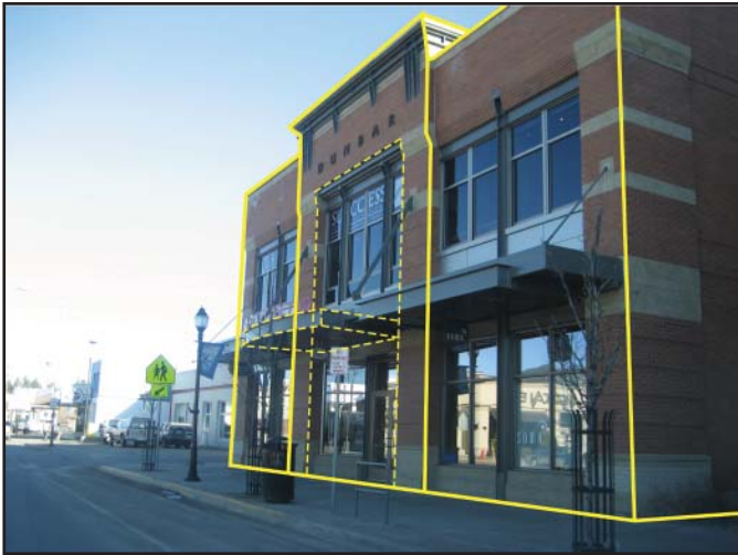
Orientation is the placement and directional relationship of the form to spaces around it. This building displays good orientation to the street, articulation and directional relationships.
